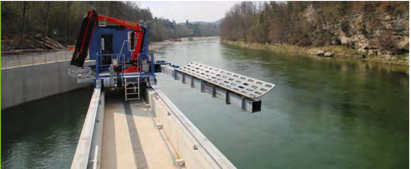
Steel construction for hydraulic engineering
